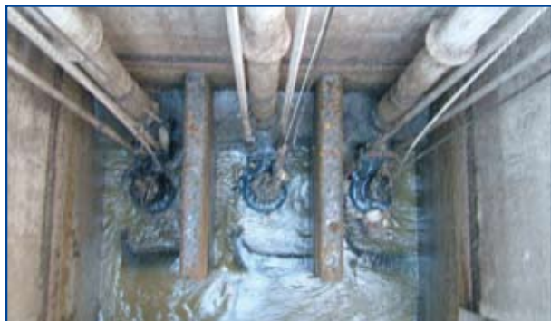
A typical prerostal installation. Note the clean sump
