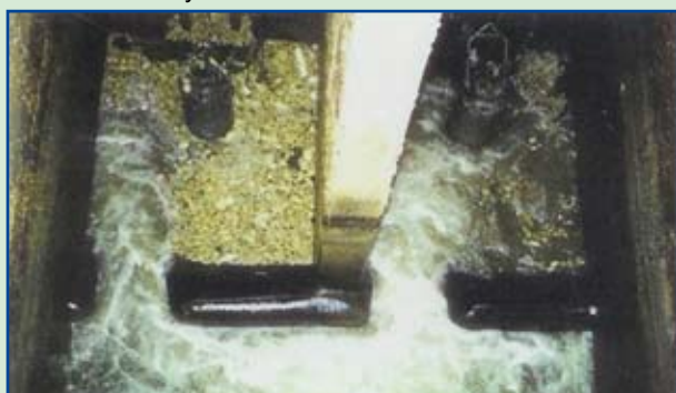
Floating material is entrained and pumped from the wet-well
